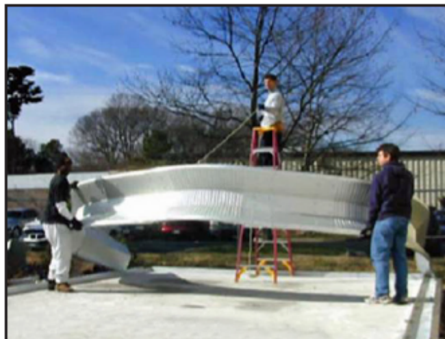
Step 2: Lift Arch & Guide with Rope
