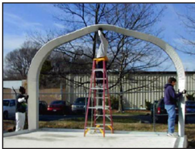
Step 4: Set Arch in Place/Secure to Foundation
