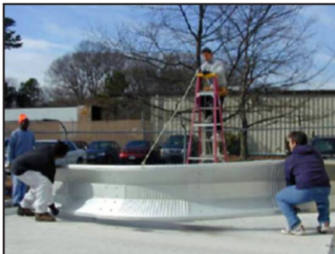
Step 1: Build Arch on the Ground
