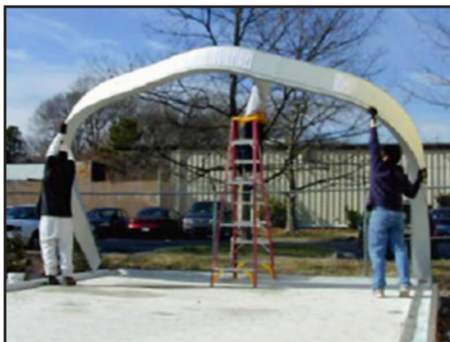
Step 3: Bring Arch to Vertical Position
